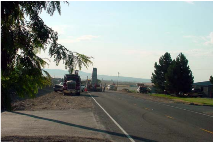
9 Loading the last pillar onto the truck
