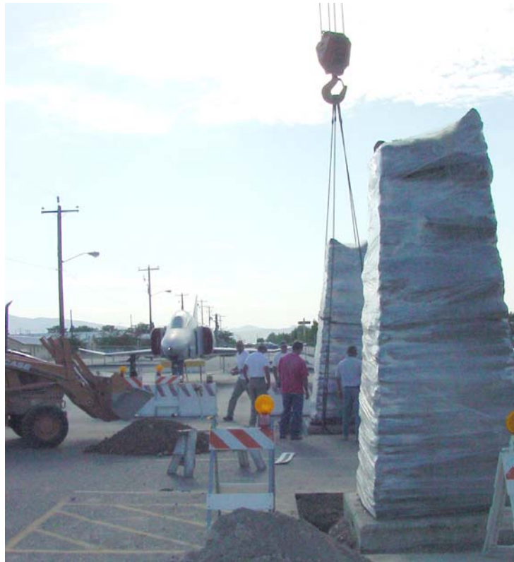
11 The last pillar is lowered into place at the Idaho Military History Museum
