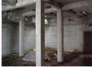
Interior of Underground Room
