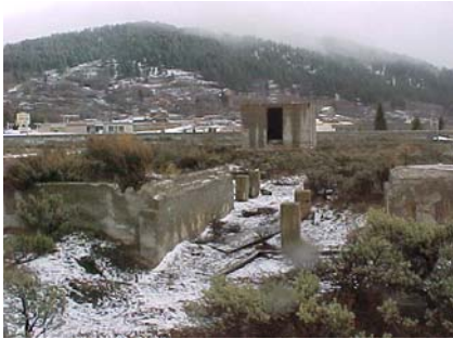
Looking East at Foundations and Paymaster Vault
