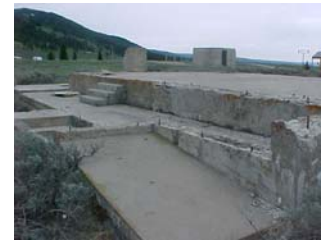
Top of Large Underground Room
